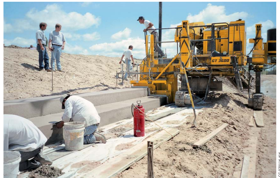
A project for 10 rows of stair-stepped risers within a new football stadium is completed in five passes around the facility with the GT-3600.
