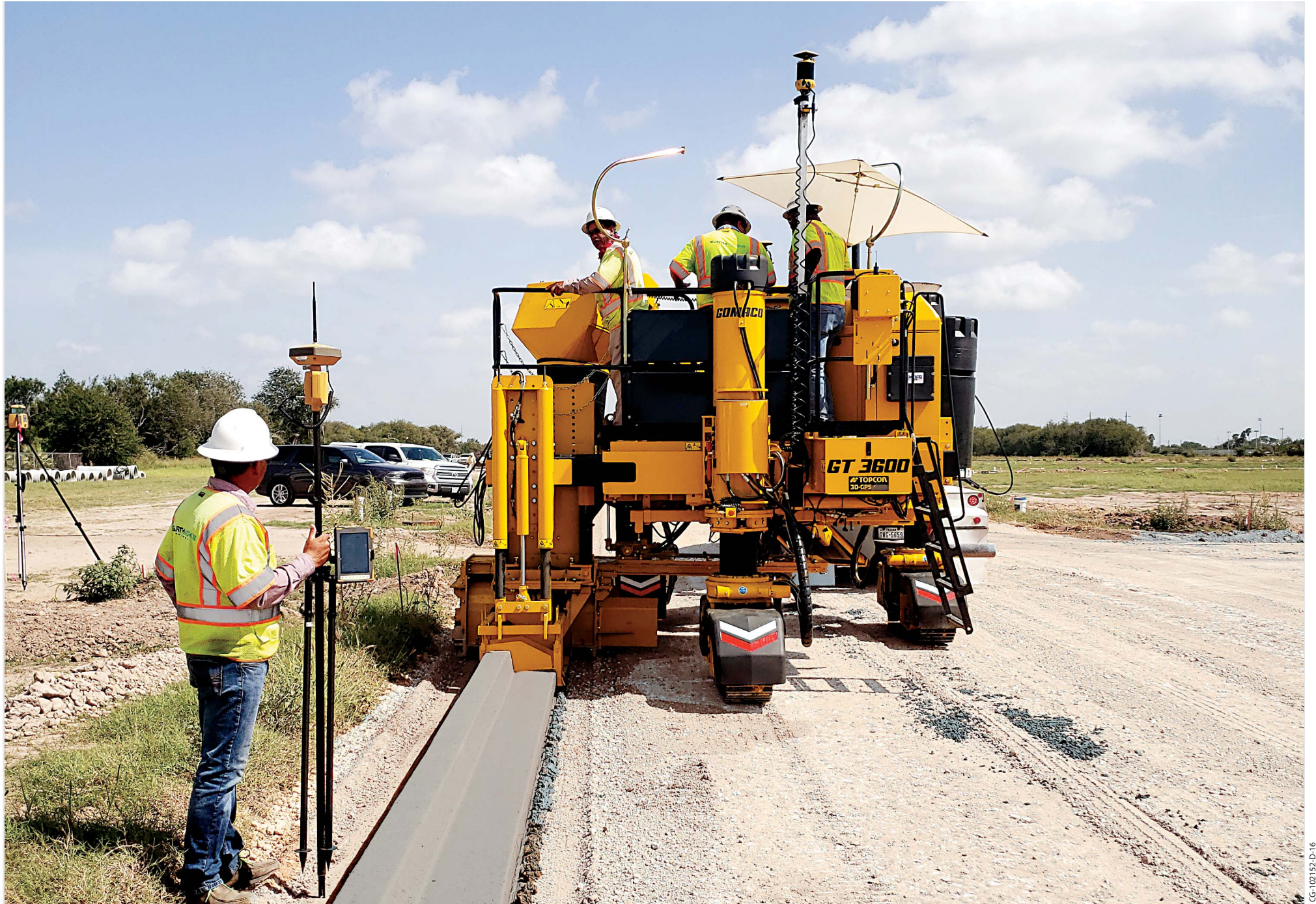
An 18 inch (457 mm) curb and gutter is slipformed using 3D machine guidance by the Xtracore GT-3600 in a new residential development.
