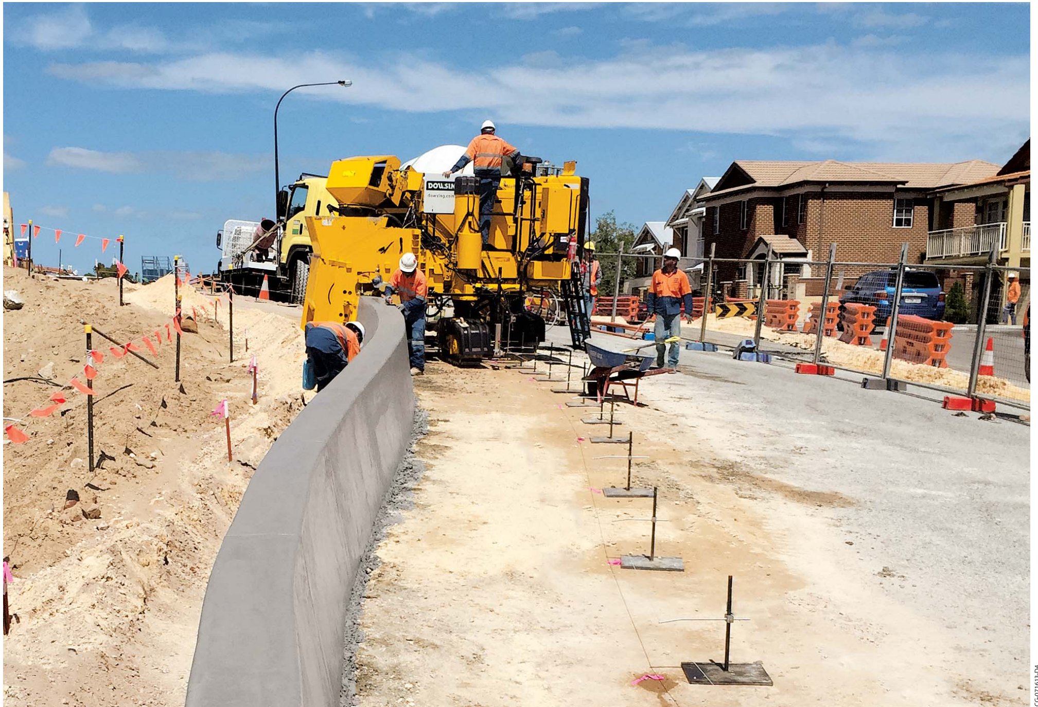
A GT-3600 slipforms variable barrier ranging in height between 34.8 to 50 inches (885 to 1270 mm) on a project in Perth, Australia.
