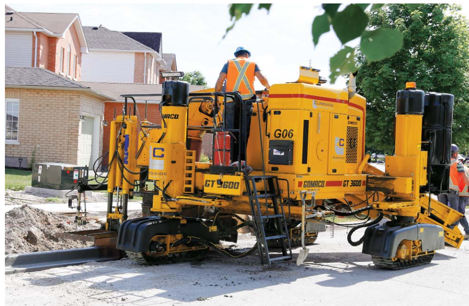
Using the telescoping mold and hold-down, the GT-3600 is able to achieve minimum clearance when slipforming curb and gutter below the existing grade in a residential area.
