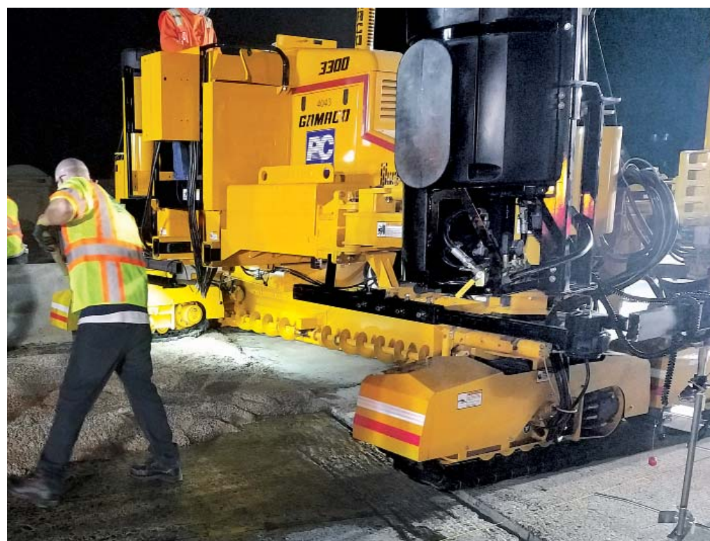
A GOMACO 3300 with a special mold paves a 0.75 inch (19 mm) thick polymer overlay on a bridge.
