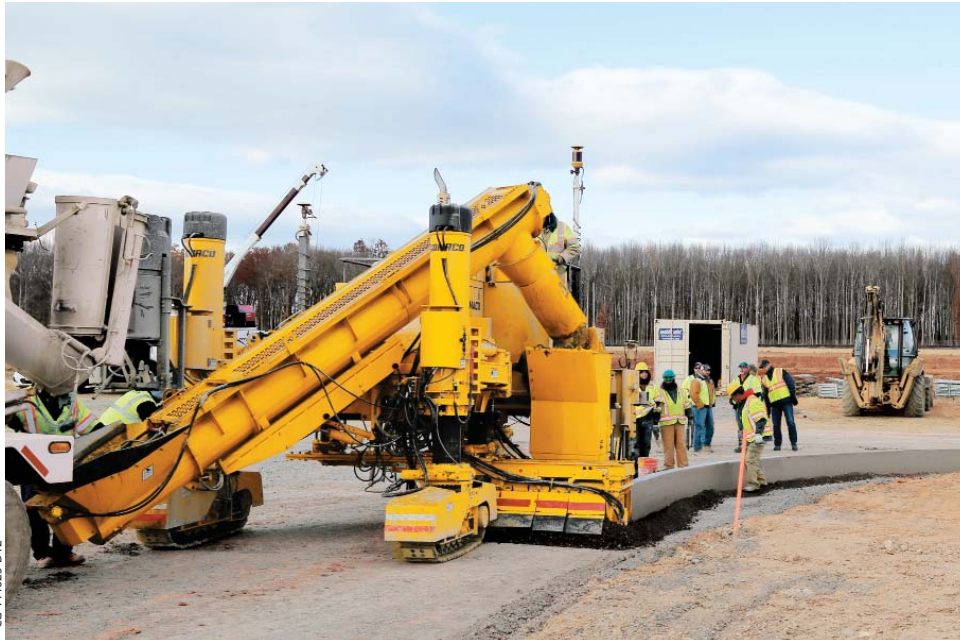
This GOMACO 3300 is equipped with a sideshifting trimmerhead and curb mold. The 3300 features the smart telescoping mold mounting system with feedback to the G+ controls for repeatable mold offset. The mold and trimmer can be hydraulically lifted over obstacles found on the job site.
