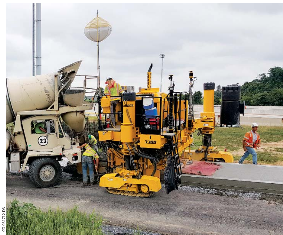
A GOMACO 3300 with an undermounted mold and 3D machine guidance slipforms a highway ramp eight feet (2.44 m) wide, 12 inches (305 mm) thick. The 3300's tracks are turned 90 degrees in the transverse position to accommodate the undermounted mold.
