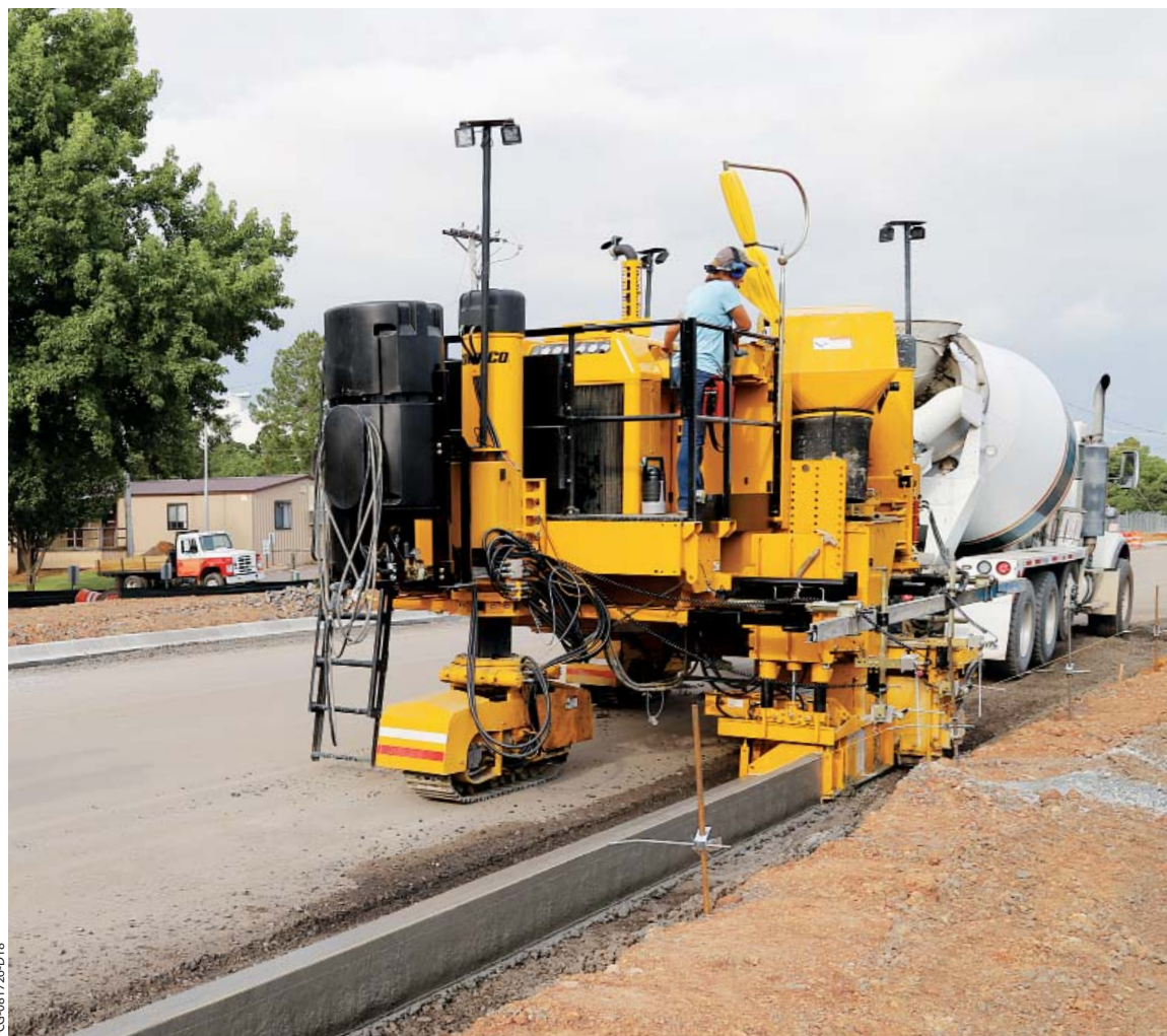
The hydraulic sideshift and lift on the 3300 allows the mold to easily slipform curb and gutter below the existing grade on rehab projects.
