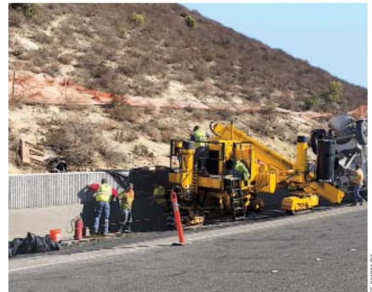
This GOMACO 3300 is slipforming a parapet wall on the left-side of the machine .
