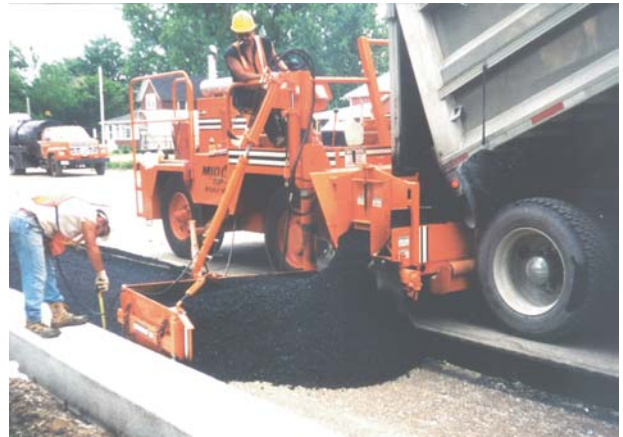
Spread binder layer below grade
