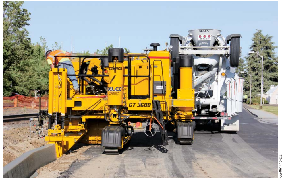
The GT-3600 slipforms stand-up curb.
