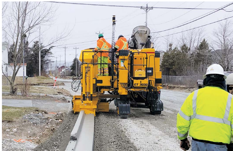
Slipforming curb and gutter in an existing residential area is done efficiently with the GT-3600 equipped with 3D machine guidance. The ability to block out existing driveways on-the-go allows for less follow up work.
