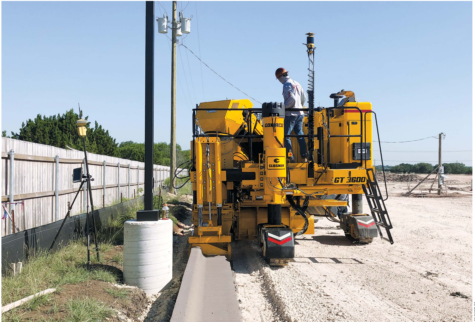
3D machine guidance helps achieve minimum clearance eliminating the need to set stringline on projects where existing utilities create challenges.
