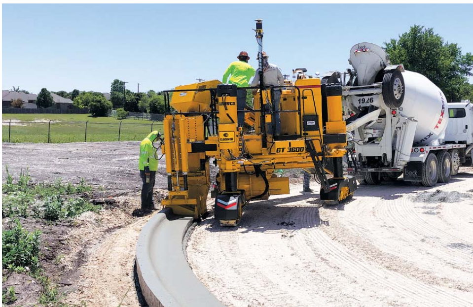
The GT-3600 trimmer features a maximum hydraulic sideshift distance of 48 inches (1219 mm), allowing the operator to slipform curb and gutter within inches of obstacles within residential areas.
