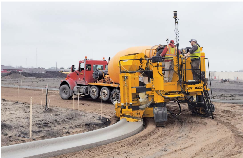
An operational speed of up to 42 feet per minute (12.8 mpm) allows for high production curb and gutter slipforming with the GT-3600.
