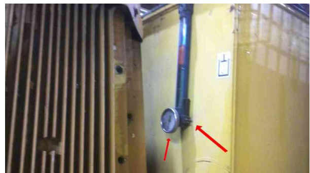
Oil level sensor not working and temperature gauge also
