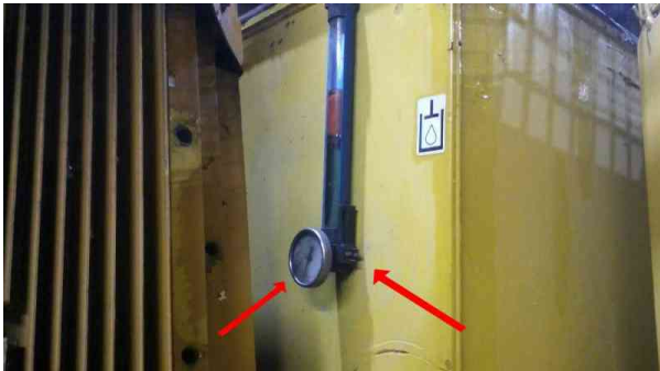
Oil level sensor and temperature gauge not working, have to be replaced
